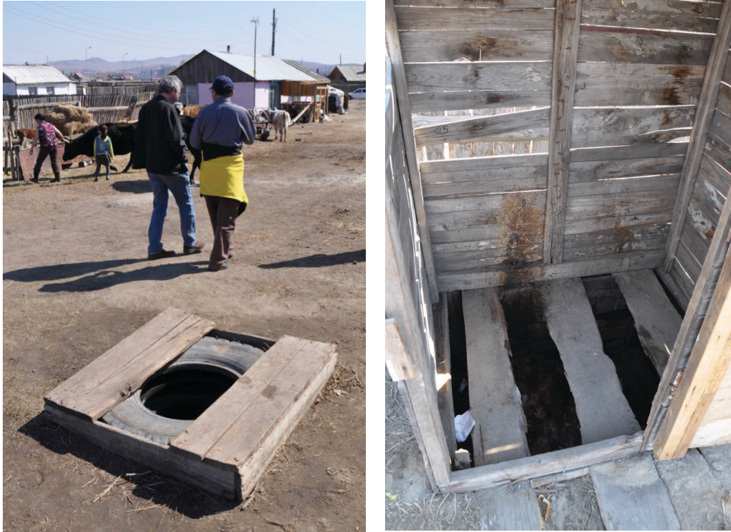
Figure 26: a.) Unprotected well accessible to cattle and b.) adjacent to typical latrine
