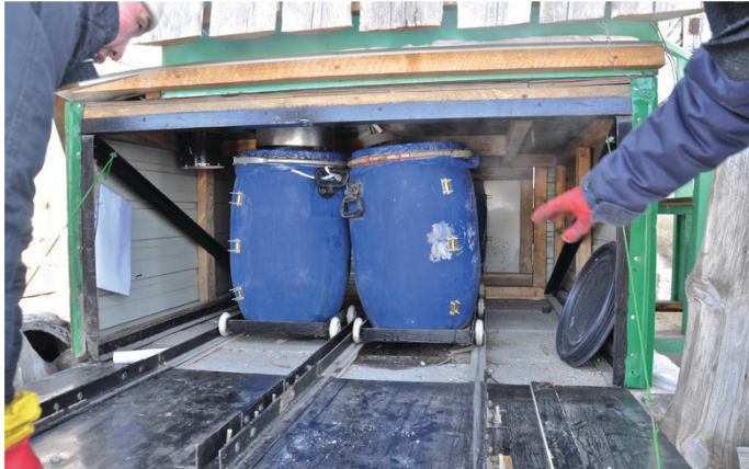
Figure 40: Container for urine and faeces accessible from roadside
